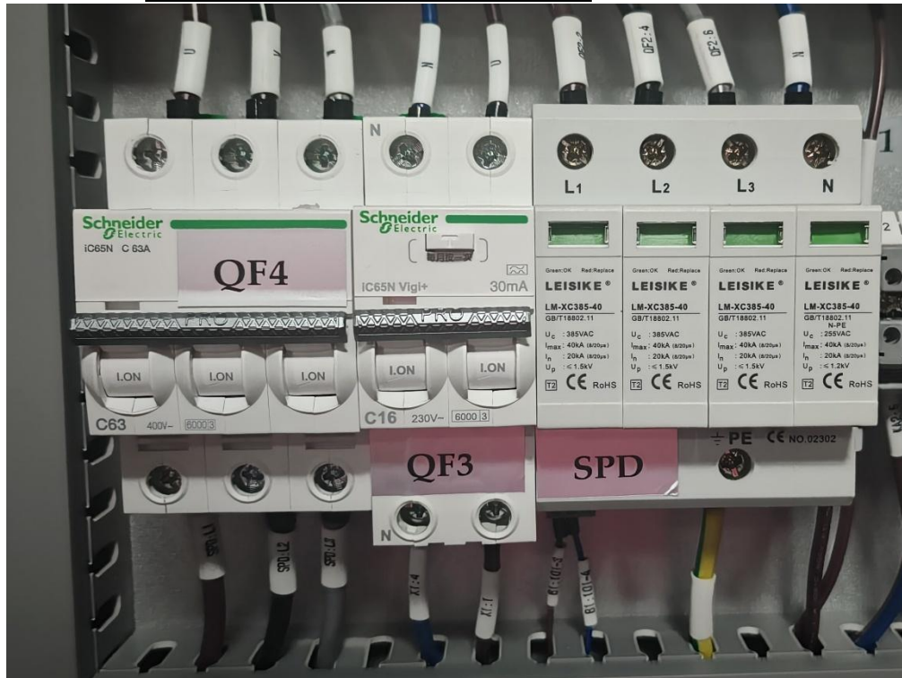
Figure 67 RCB, MCB and SPD
