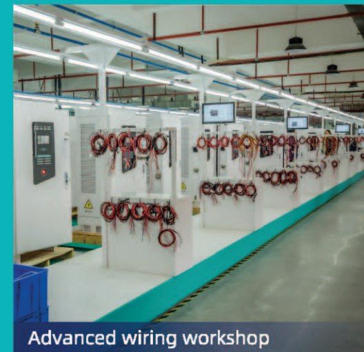
Advanced wiring workshop
